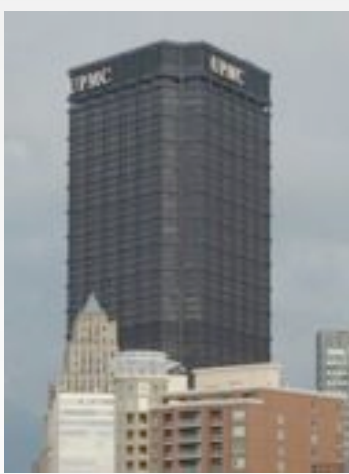
The USX Tower, the iconic home US Steel, now sports the UPMC logo on the top floors of the building.
